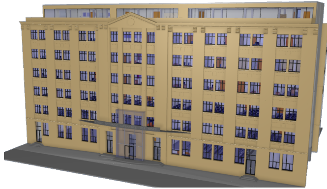
Figure 3: Espace Fauriel Building of Mines Saint-Étienne
